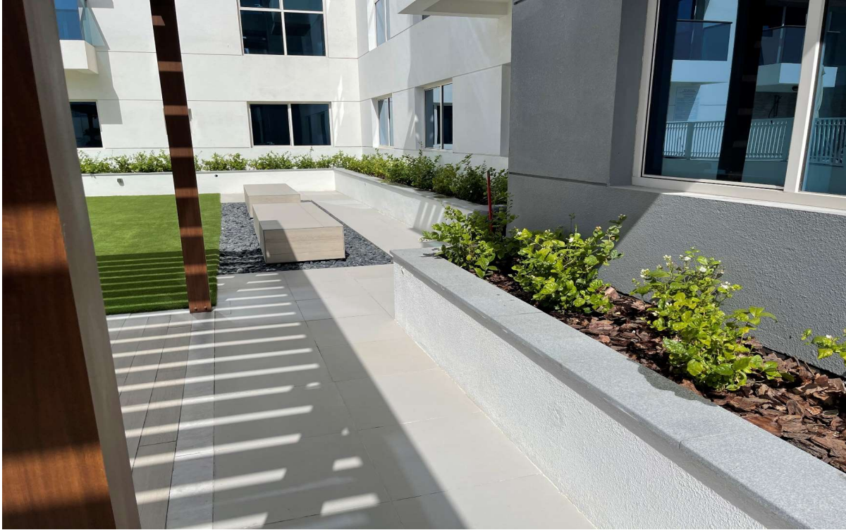
Tiling work at JVT in Residential Tower
