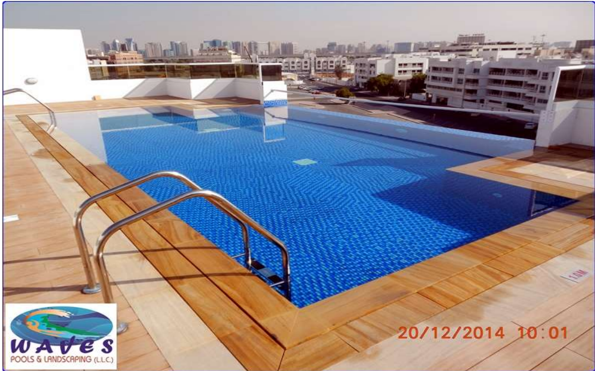
Overflow Pool at Al Karama in Residential tower. Client : WASL LLC
