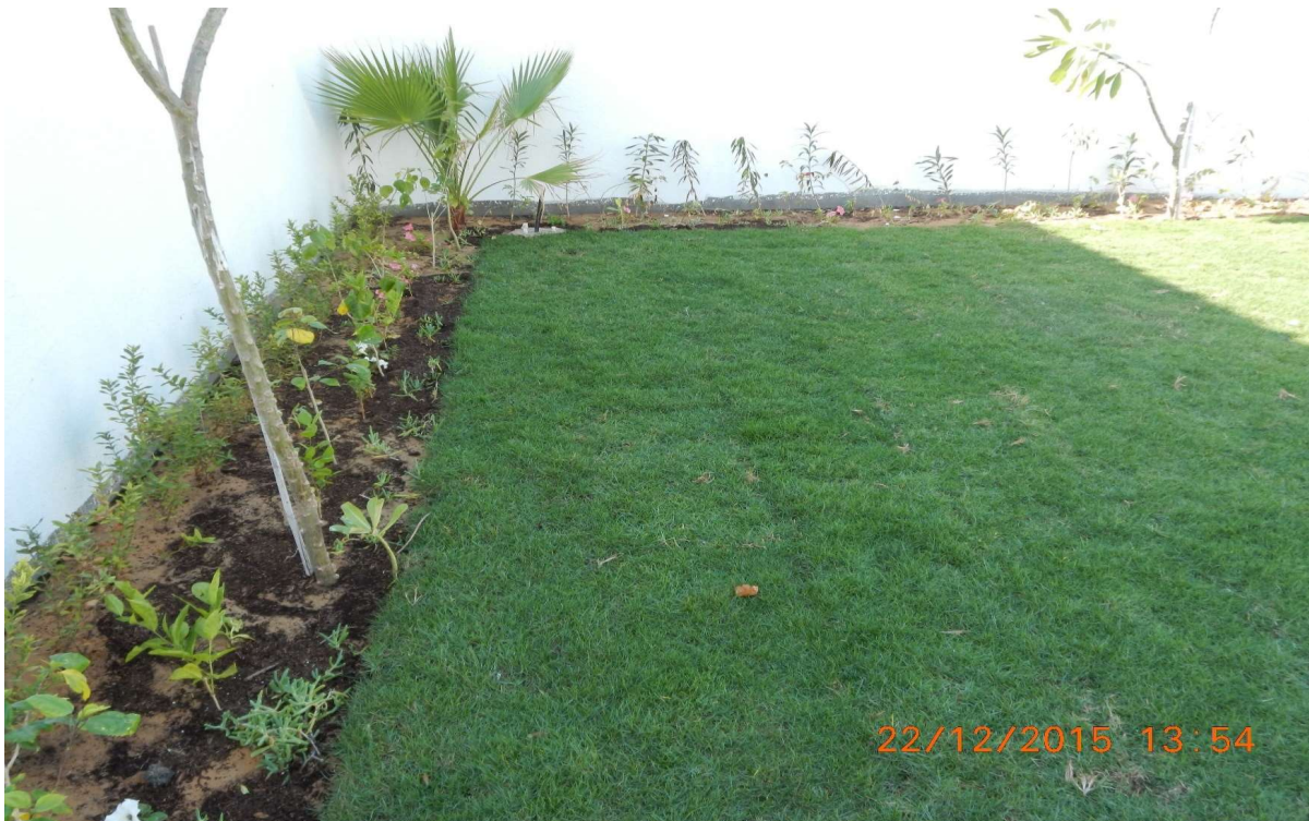
Landscaping work at Ajman in Private Villa.
