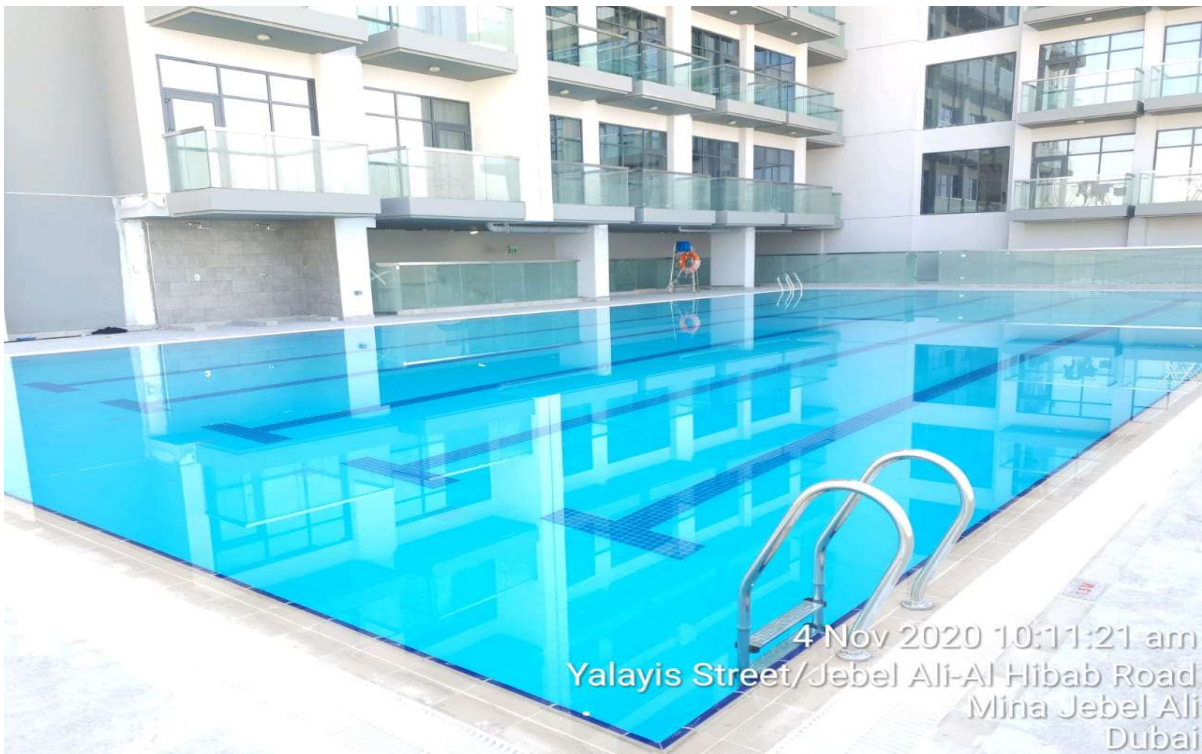
Overflow Pool at Al Furjan in Residential Tower
