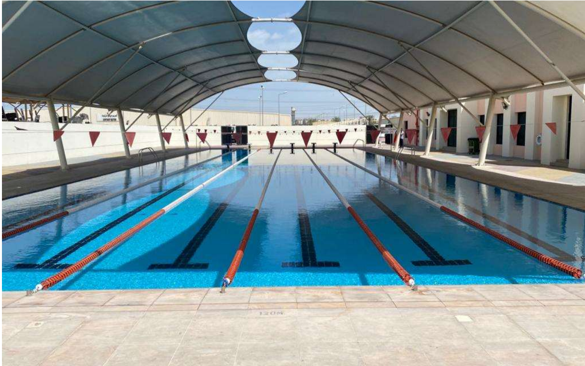
Olympic Pool at Silicon Oasis. Client - Dubai Police
