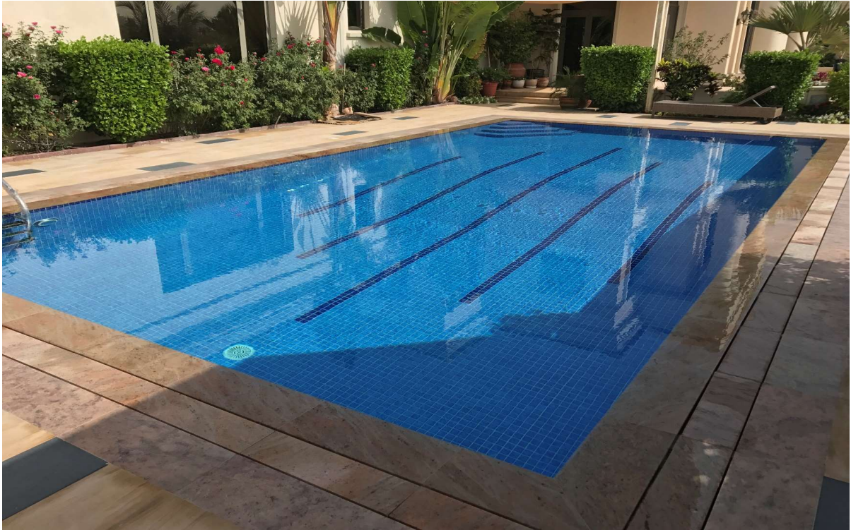
Overflow Pool at Palm Jumeirah in Private Villa.
