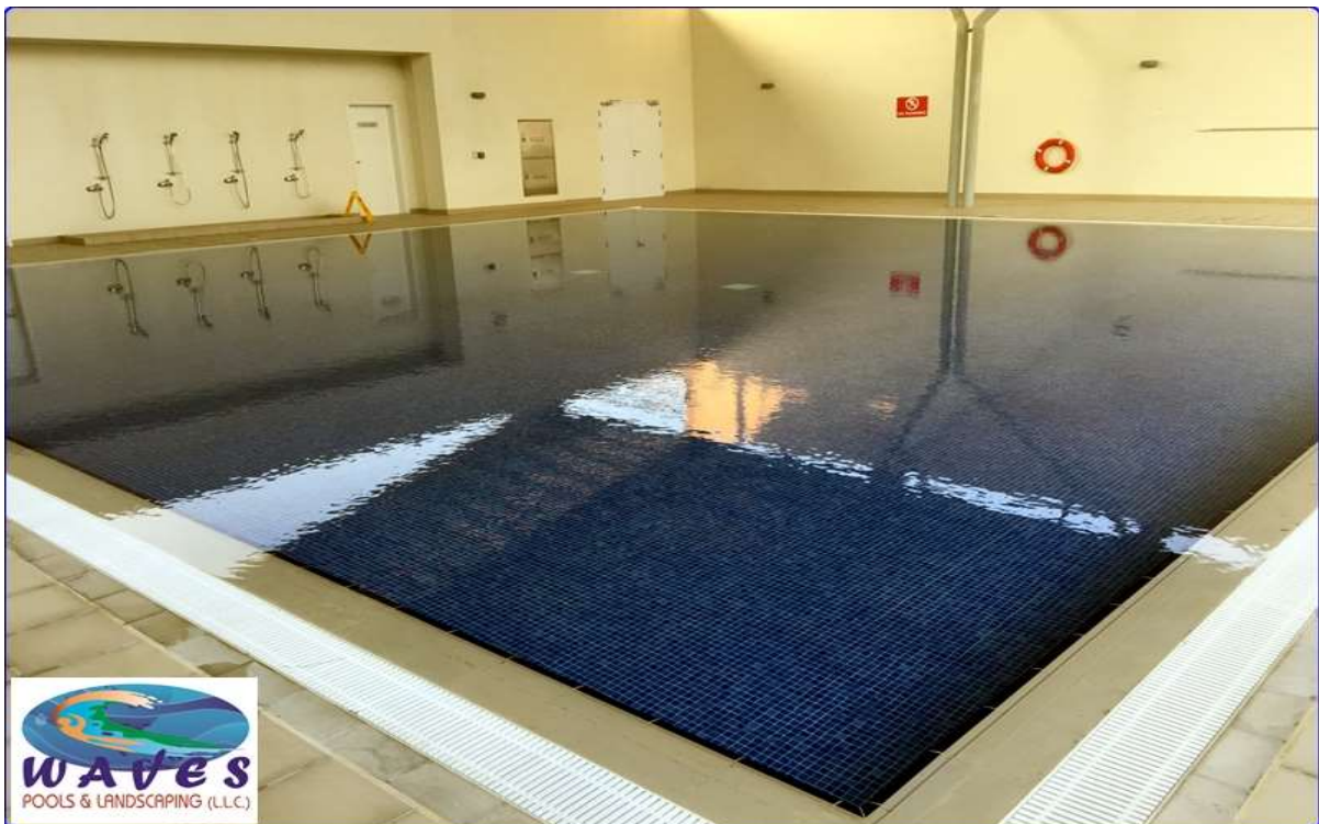
Overflow Pool at Nad Al Hamar in King's School
