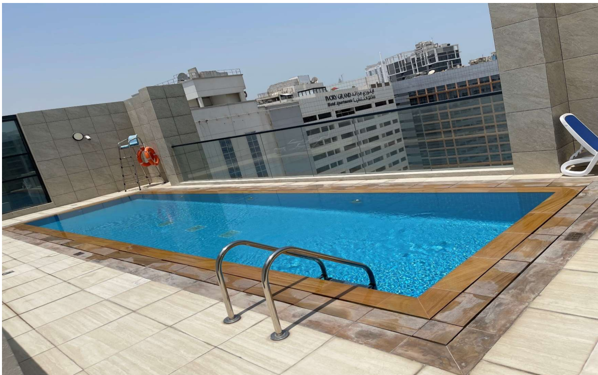
Overflow Pool at Al Barsha in Residential Tower
