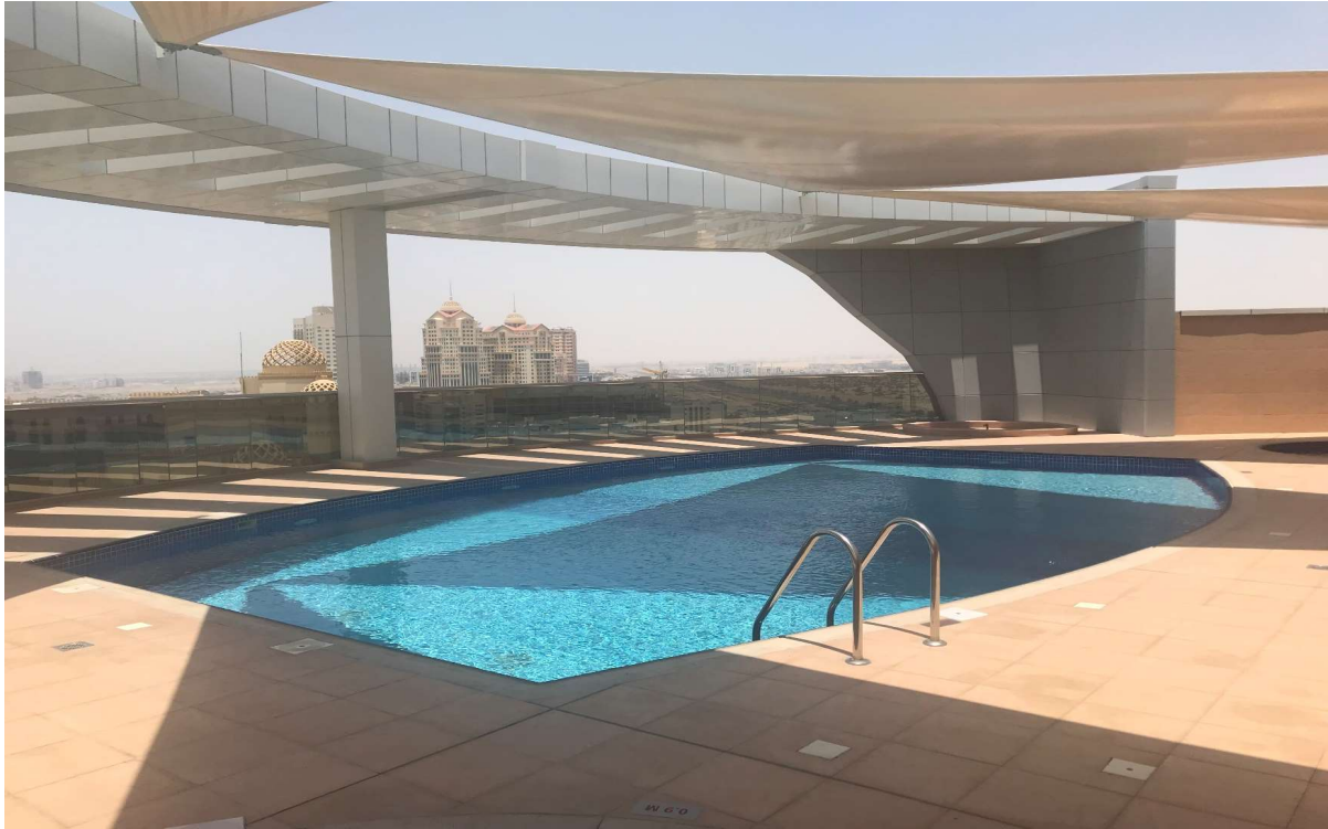
Skimmer Pool at Dubai Silicon Oasis in Residential Tower
