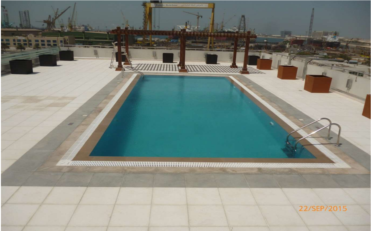
Overflow Pool at Port Rashid in Hotel Building. Client - WASL LLC
