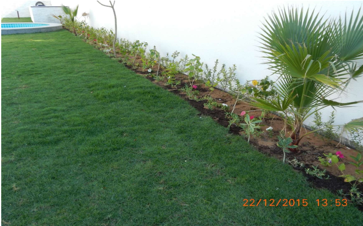
Landscaping work at Ajman in Private Villa.
