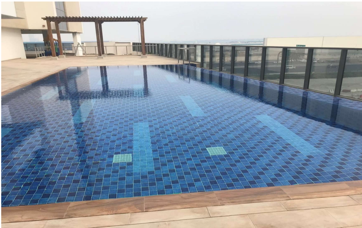
Infinty Pool at Al Jaddaf in Residential Tower
