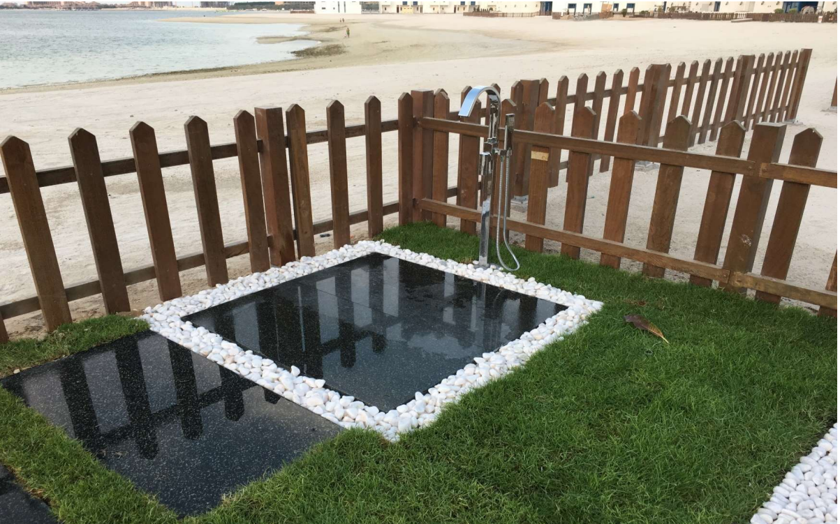
Landscaping work at Palm Jumeirah in Private Villa.
