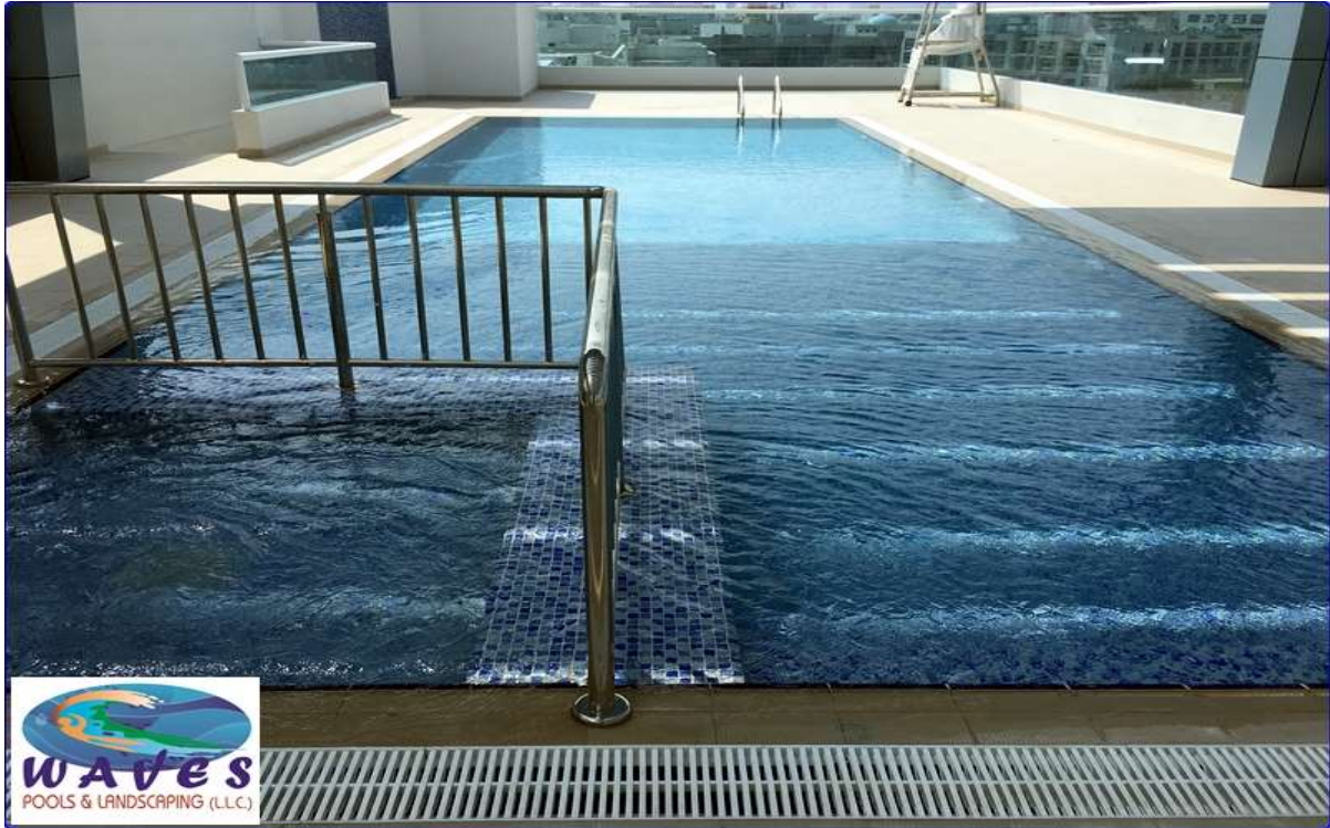
Overflow Pool with Kid's Pool at Al Karama in residential Tower. Client - WASL LLC
