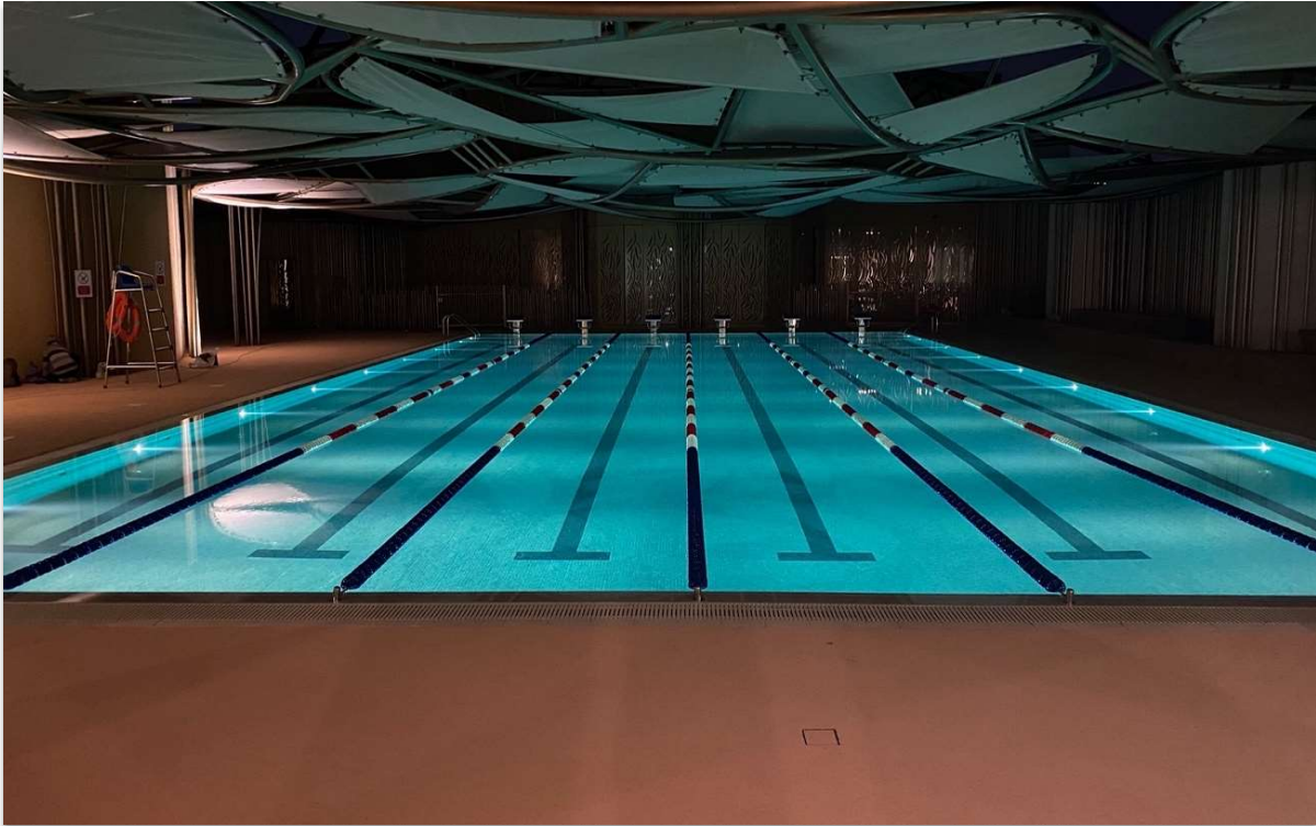
Overflow Pool at Al Khawaneej in Al Marafa School.
