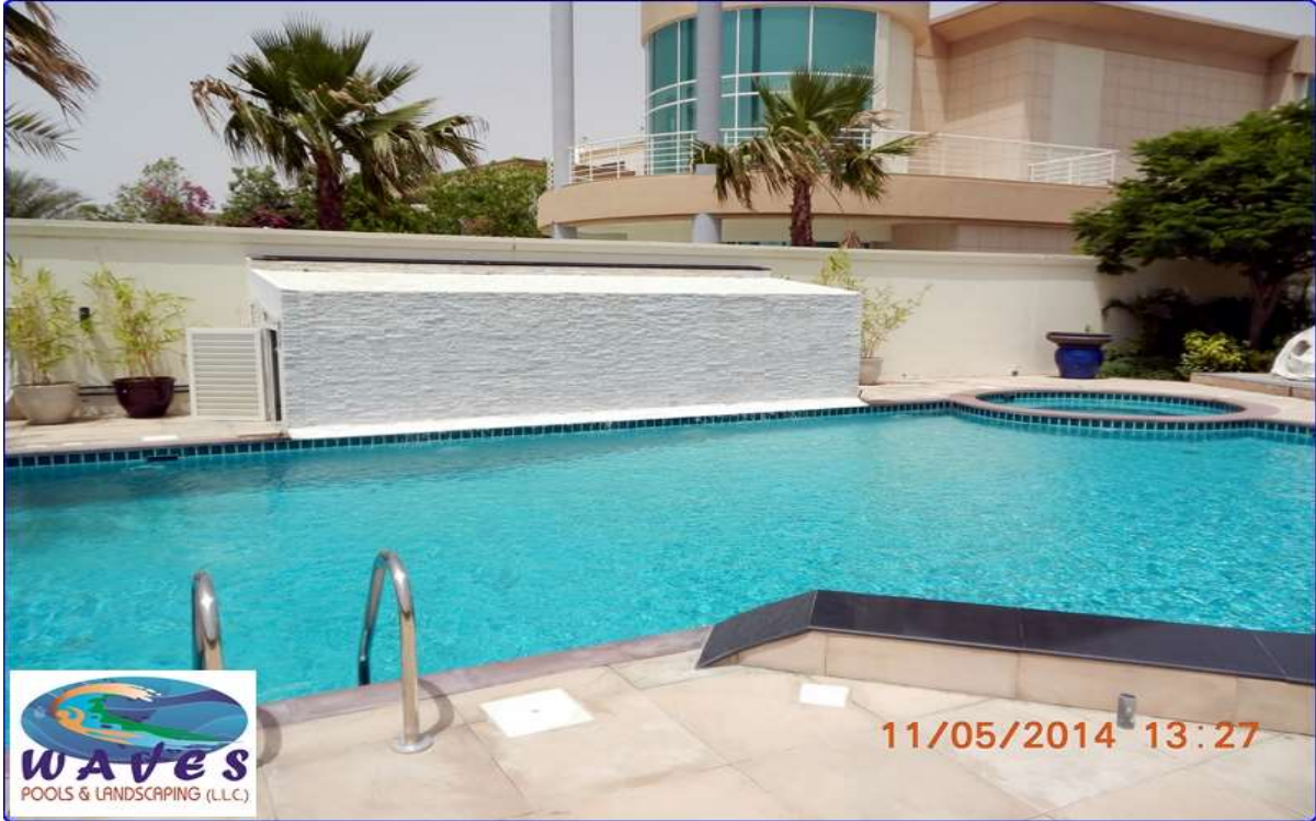
Overflow Pool with Jacuzzi at Emirates Hills in Private Villa.
