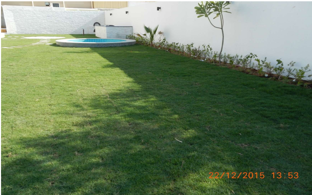
Landscaping work at Ajman in Private Villa.
