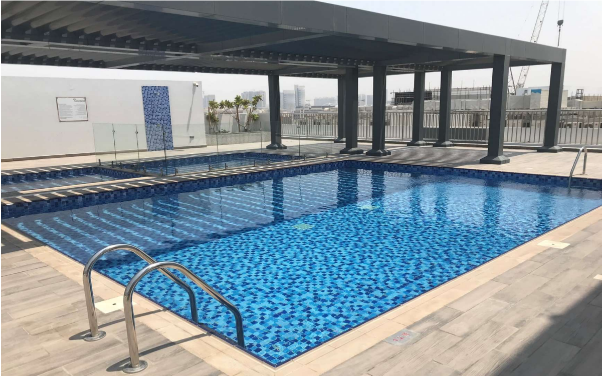
Overflow Pool at Port Rashid in Residential Tower : Client - WASL LLC
