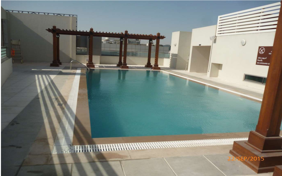
Overflow Pool at Deira in Hotel Building. Client - WASL LLC
