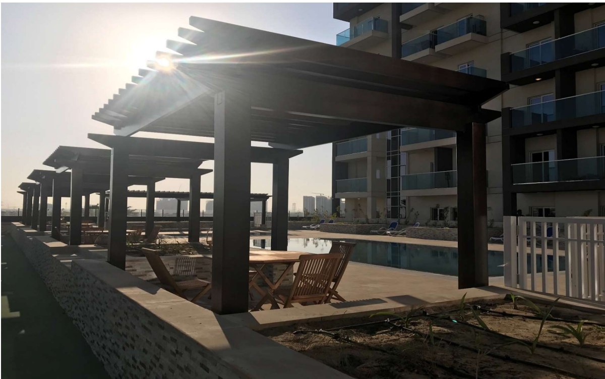
Pergola at Al Furjan in Residential Tower
