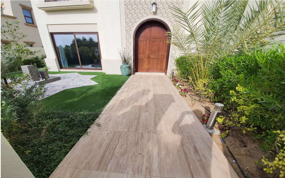
Landscaping & Tiling work at Arabian Ranches 3rd in Private Villa
