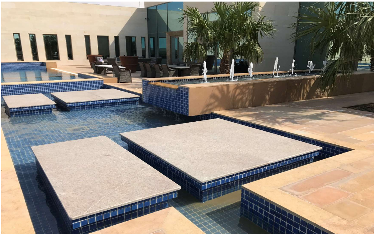
Overflow Pool with Water Body at Nad Al Sheeba in Private Villa
