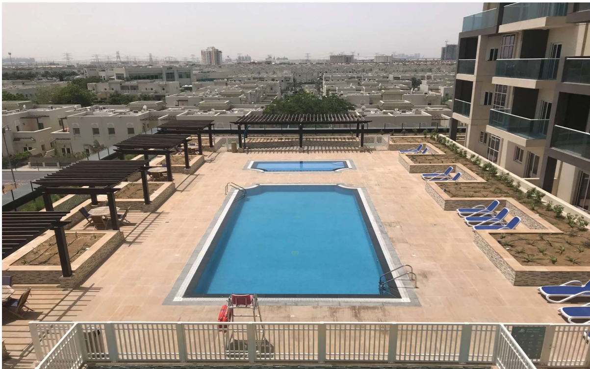
Overflow Pool with Kid's Pool at Al Furjan in Residential Tower
