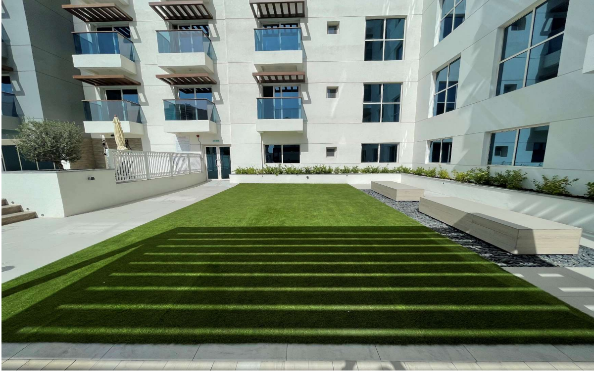
Artificial Grass work at JVT in Residential Tower
