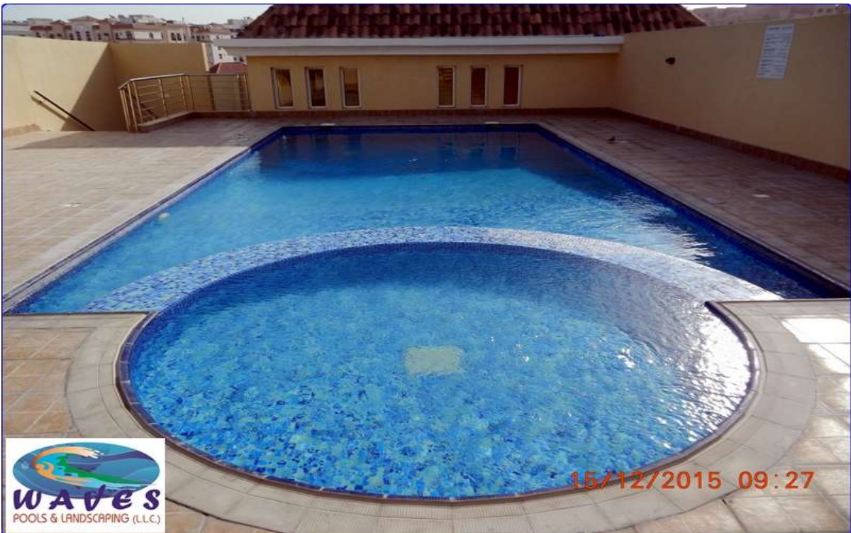
Overflow Pool at Al Jaddaf in Residential Tower.
