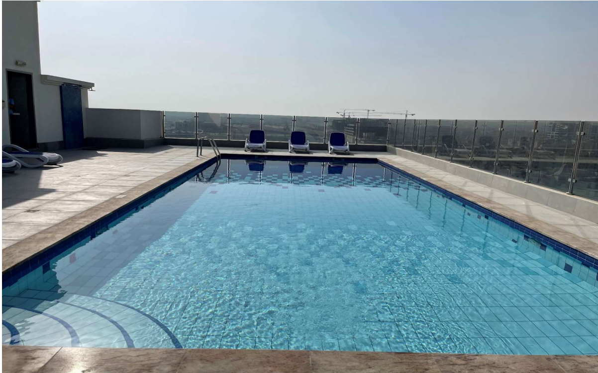
Skimmer Pool at International City in Residential Tower
