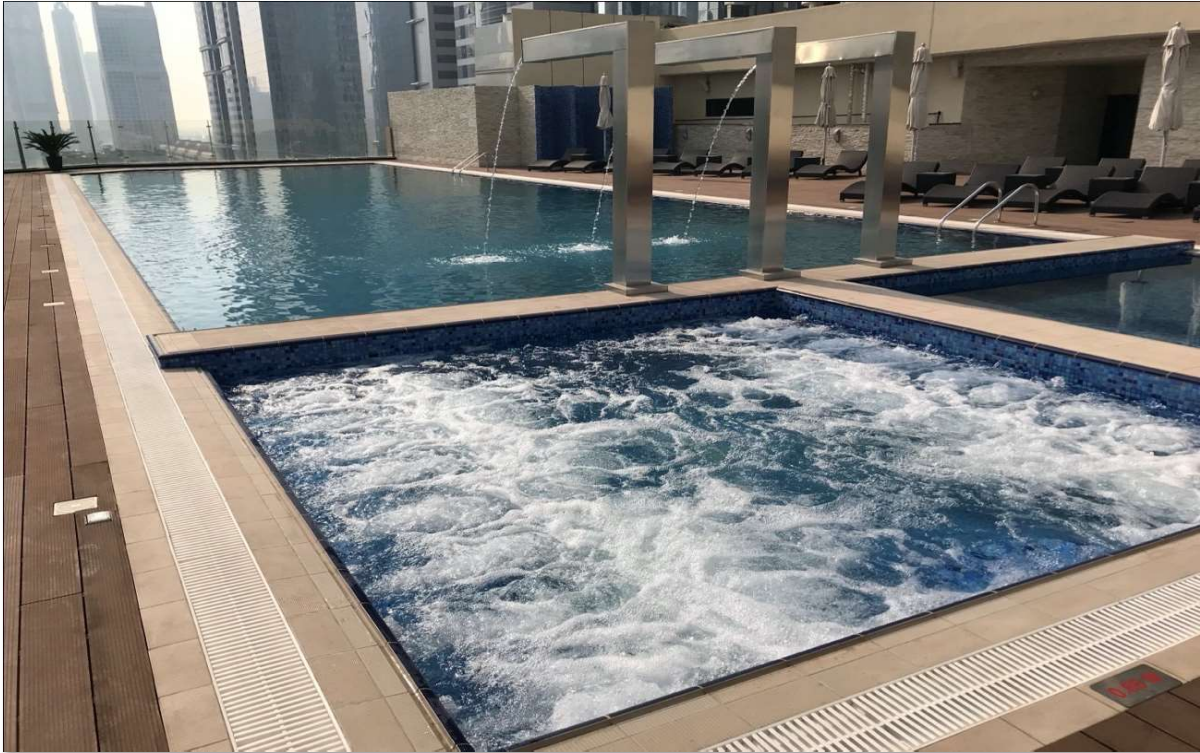
Overflow Pool with Kid's Pool at GEVORA Hotel - World Tallest Tower
