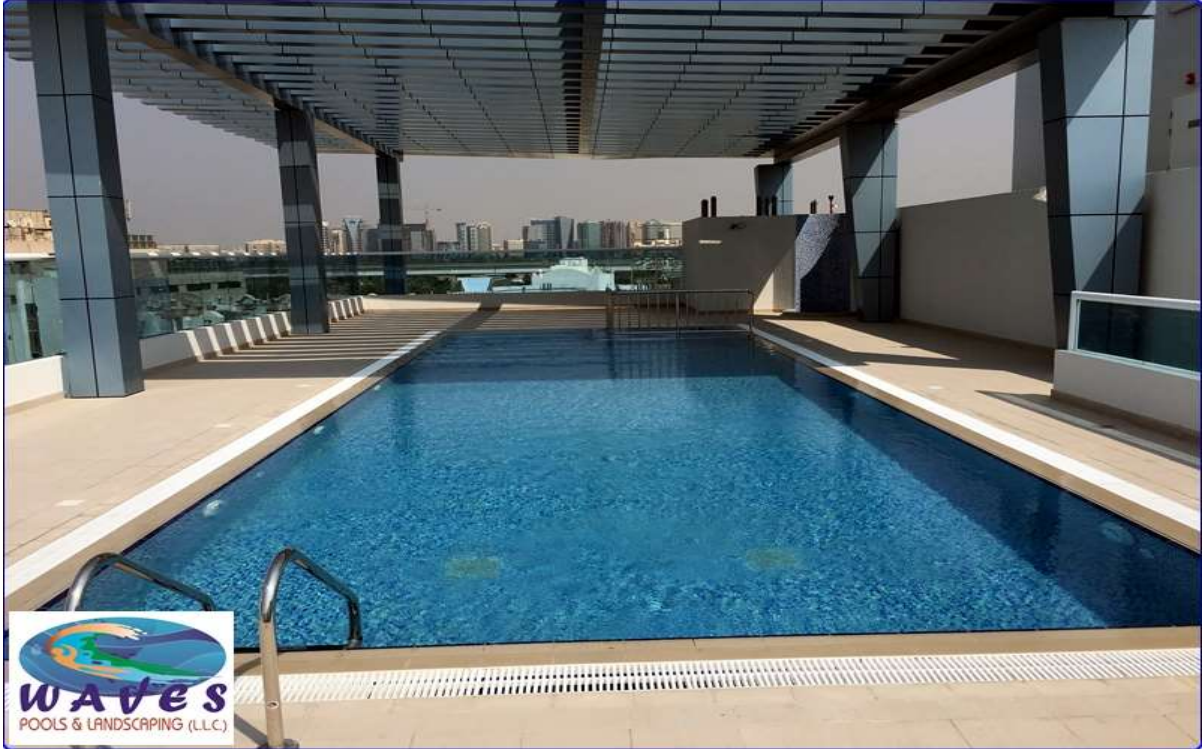
Overflow Pool with Kid's Pool at Al Karama in residential Tower. Client - WASL LLC
