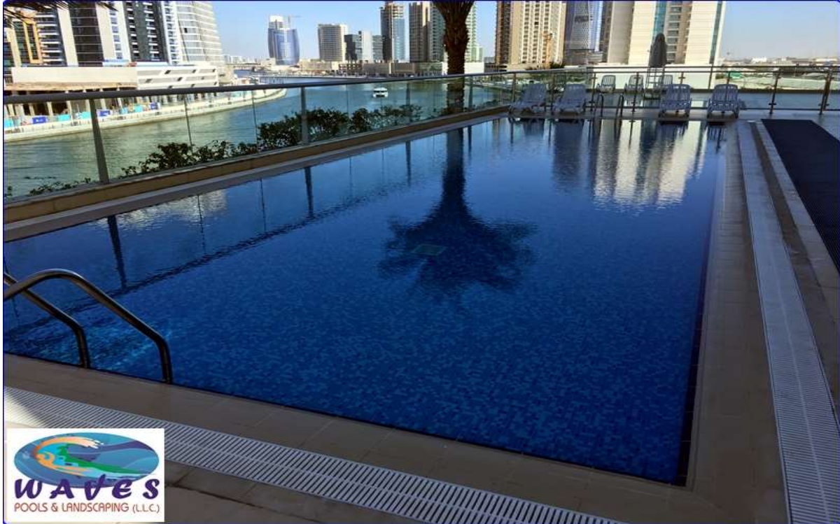
Overflow Pool with Kid's Pool at Business Bay - Client : M/s. Deyaar Developments PJSC
