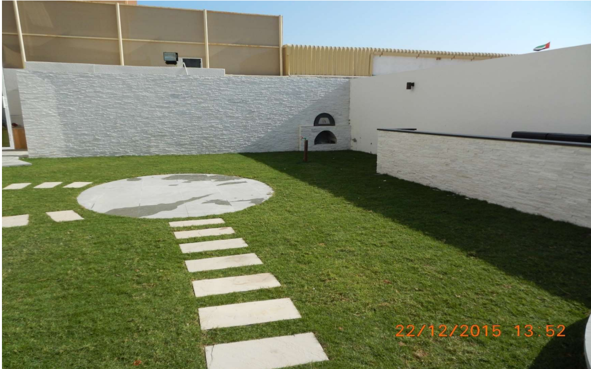
Landscaping work at Ajman in Private Villa.
