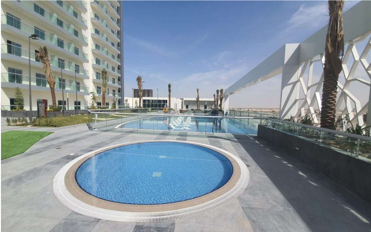
Kid's Pool at Residential Tower at Al Barsha, Client : Deyaar Developments PJSC
