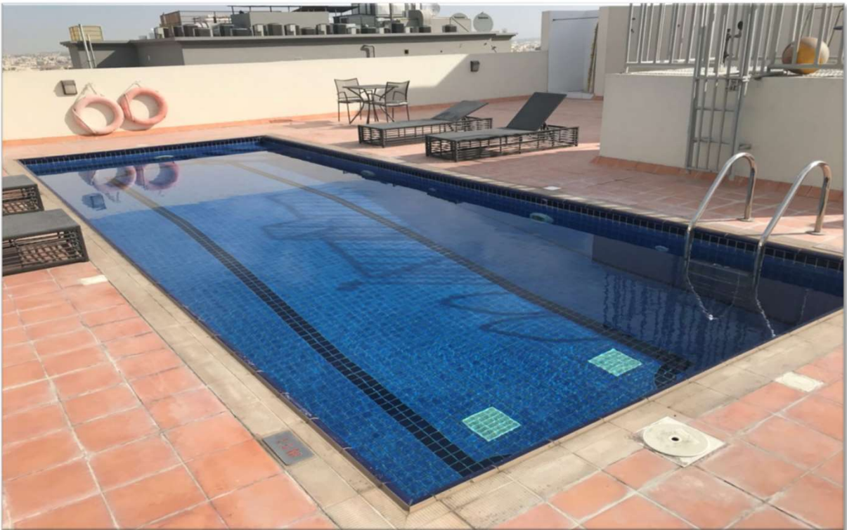
Overflow Pool at Silicon Oasis in Residential Tower
