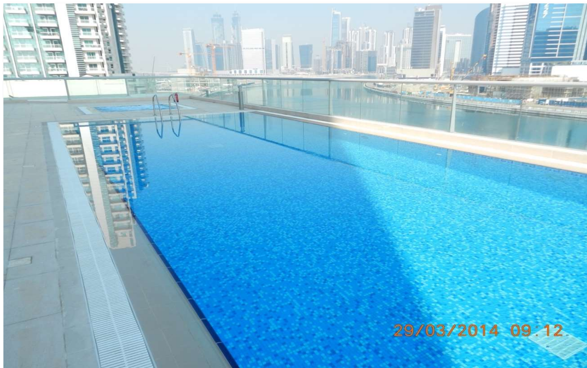
Overflow Pool with Kid's Pool at Business Bay - Client : M/s. Deyaar Developments PJSC
