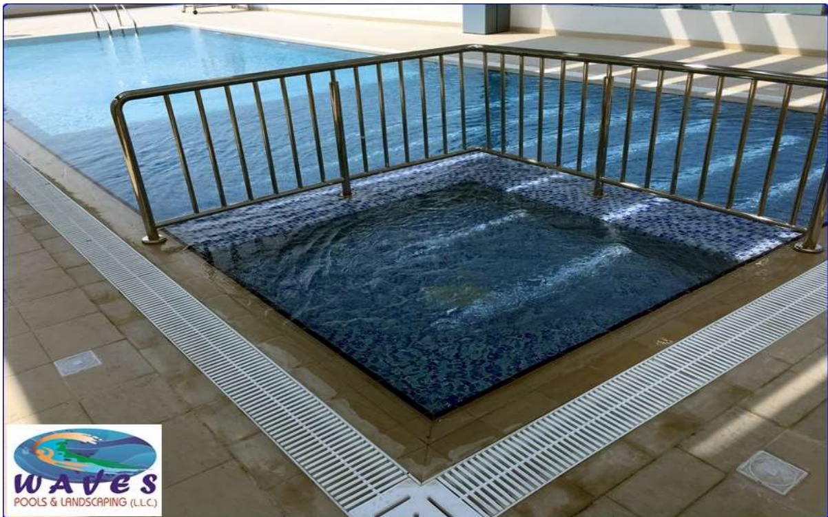
Overflow Pool with Kid's Pool at Al Karama in residential Tower. Client - WASL LLC
