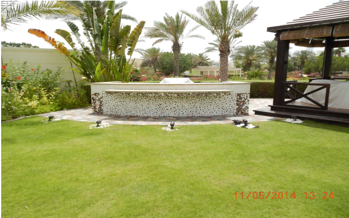
BBQ & Landscaping work at Emirates Hills in Private Villa.
