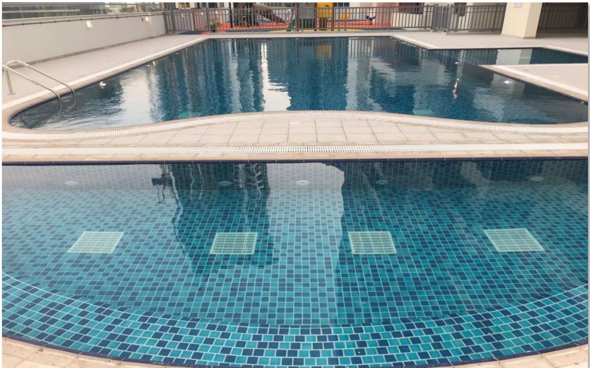
Overflow Pool with Kid's Pool at Bhawan Tower at Business Bay.
