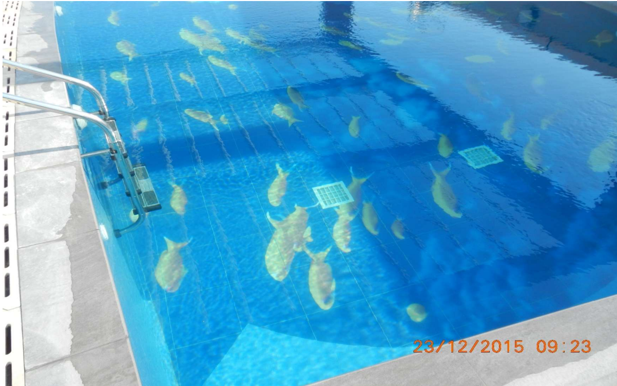
Overflow Pool at Al Muhasiana in Residential Tower.
