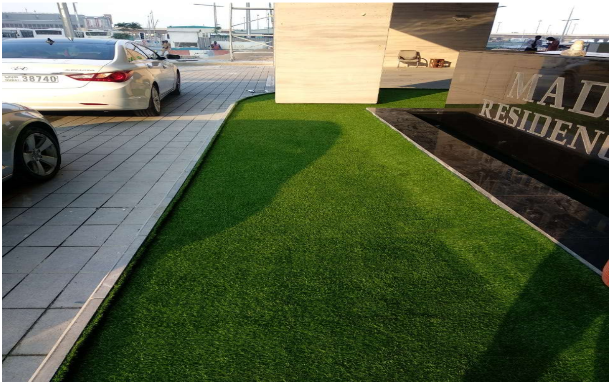
Artificial Grass work at Business Bay in Residential Tower
