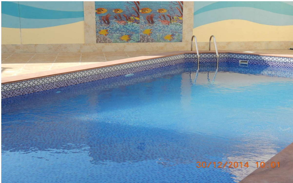
Skimmer Pool at Mirdiff in Private Villa
