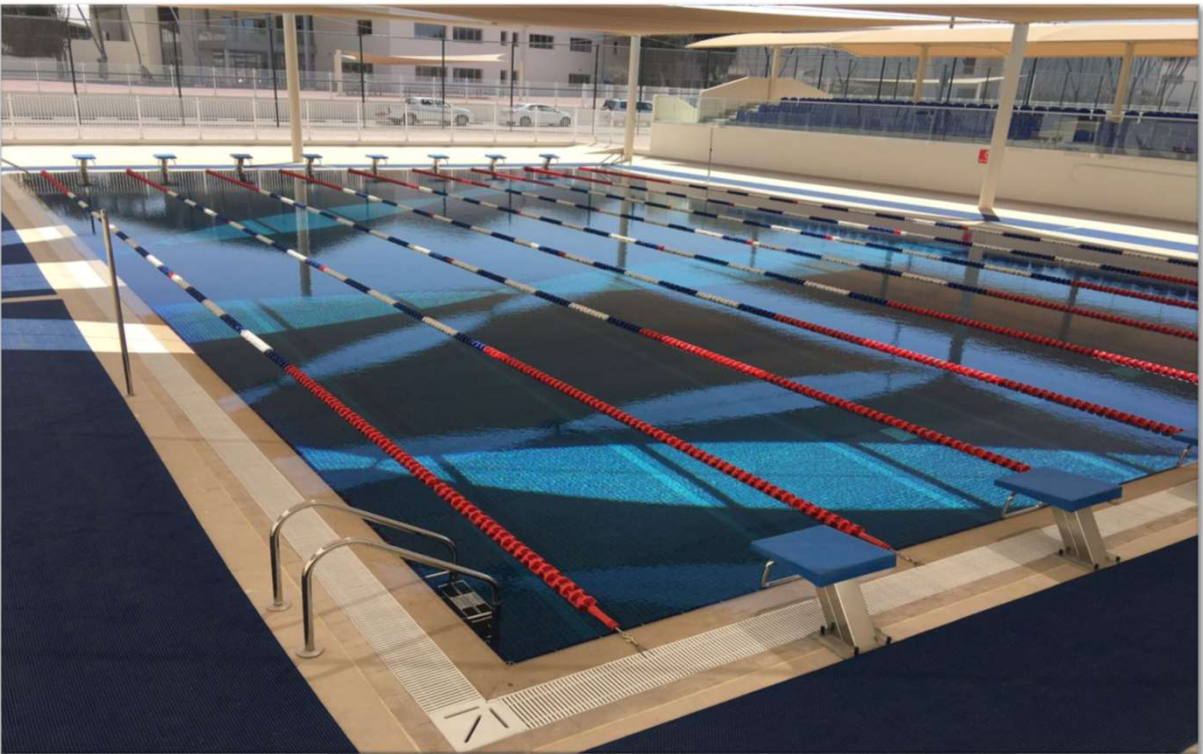
Training Pool at Al Barsha in King's School
