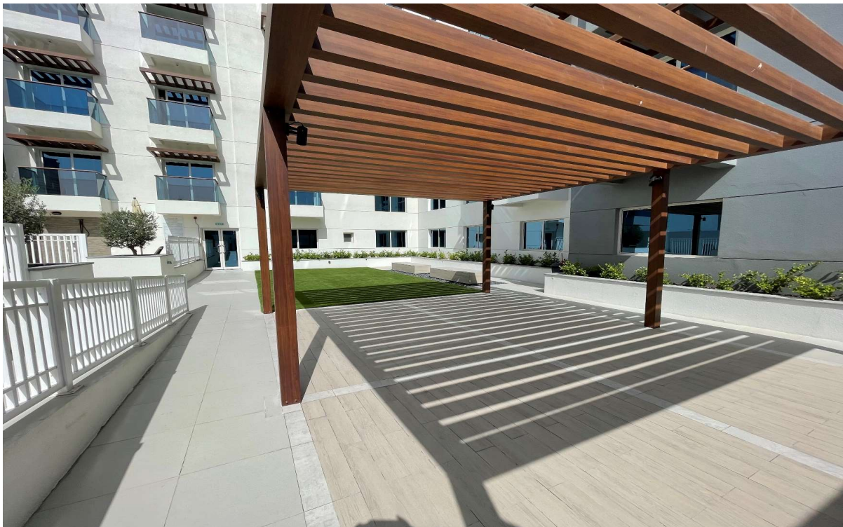
Tiling work at JVT in Residential Tower
